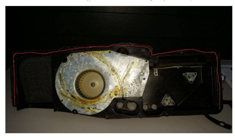
Step 11: Continue to install the rest of the foam gaskets and reassemble the box.
